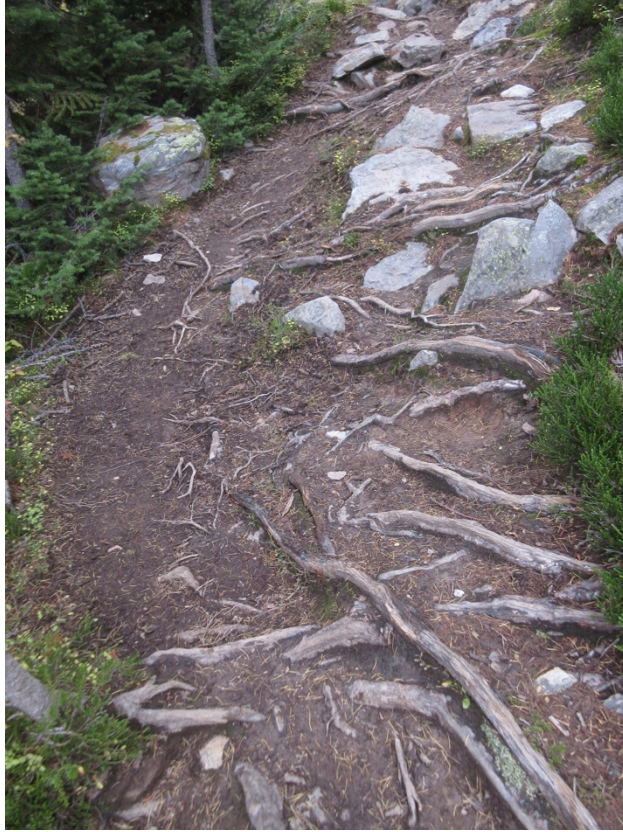
Side slope migration on Upper Big Larches trail
