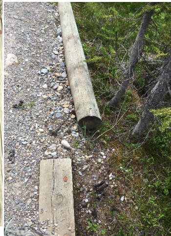
Turnpike failure on Opabin Plateau
