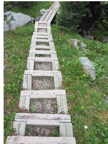
Inappropriate timber construction, Opabin
