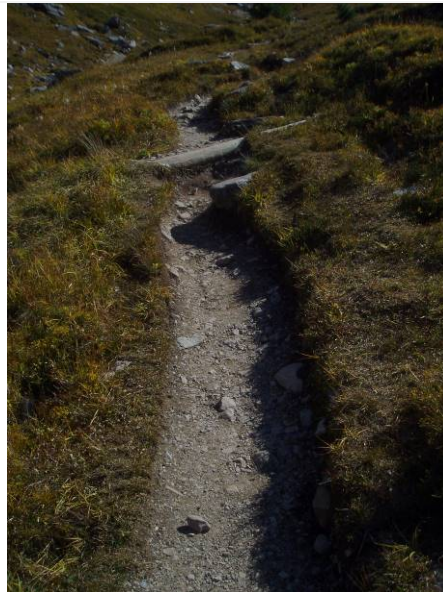
Example of water bar repairing water running along trail
