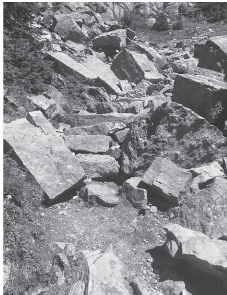
Boulders moved, new steps built!
